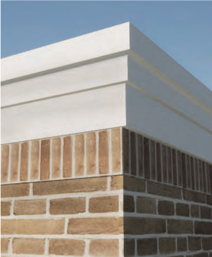
RENDER OF GFRC CORNICE, BRICK SOLDIER COURSE AND BRICK IN RUNNING BOND PATTERN W/ FLEMISH BOND EVERY 13 COURSES
