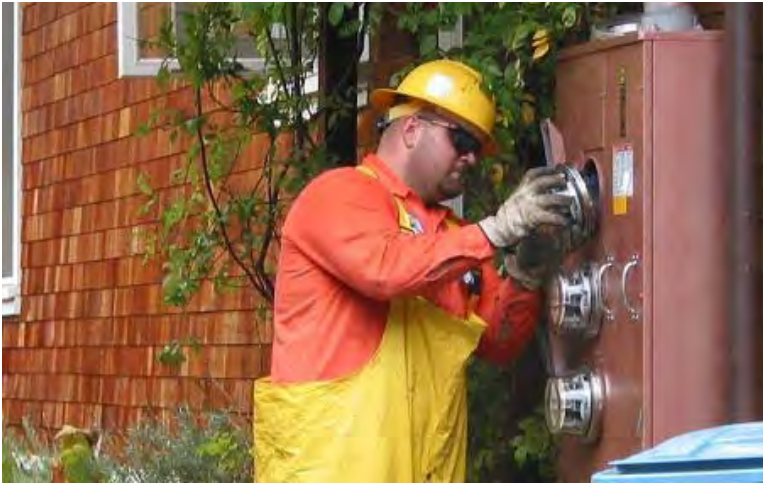
Electric Troubleshooter installing an electric meter to provide service to a customer
