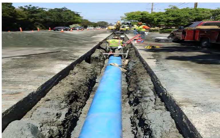
Installed 16" HDPE pipe waiting to be backfilled
