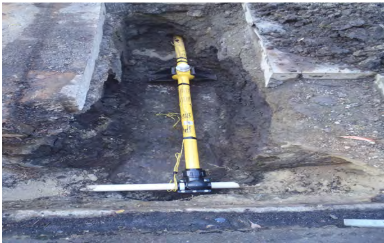
Installed HDPE gas service pipe
