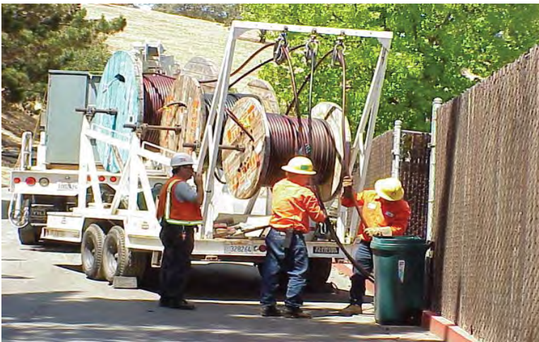
Electric crews installing new underground cables
