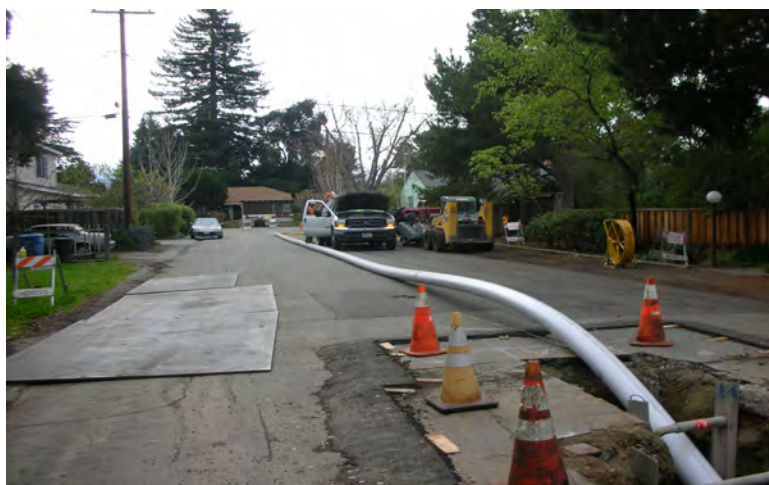
Trenching for installation of HDPE sewer main by directional drilling method
