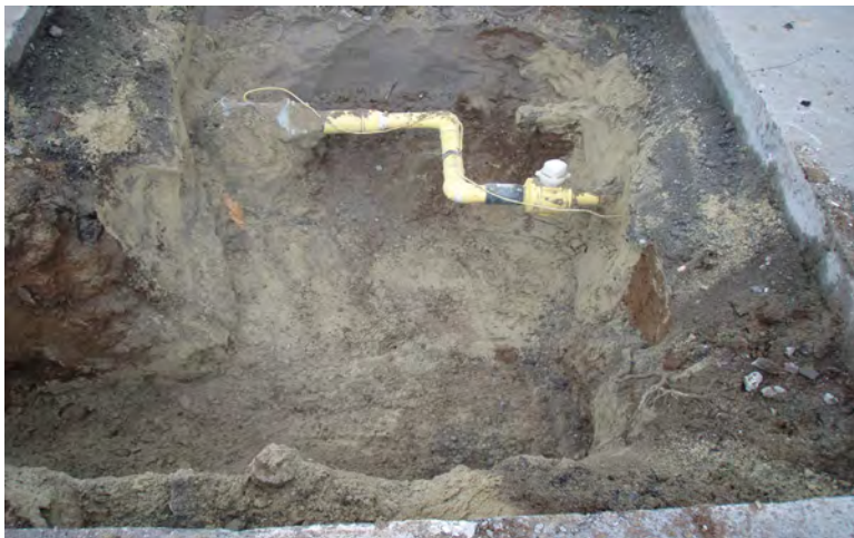
Installation of new HDPE gas service main
