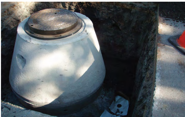
Sewer manhole base
