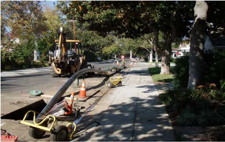
Installation of 8" HDPE pipe by directional drilling method
