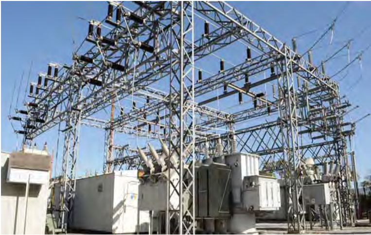
Electric Substation transformer and bus structure
