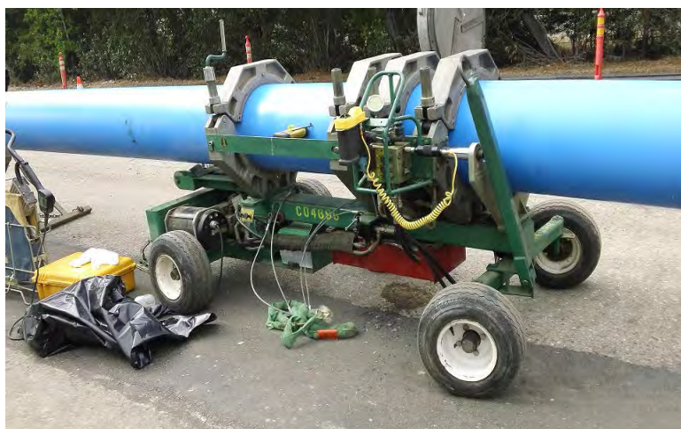
16" HDPE pipe being fused prior to installation
