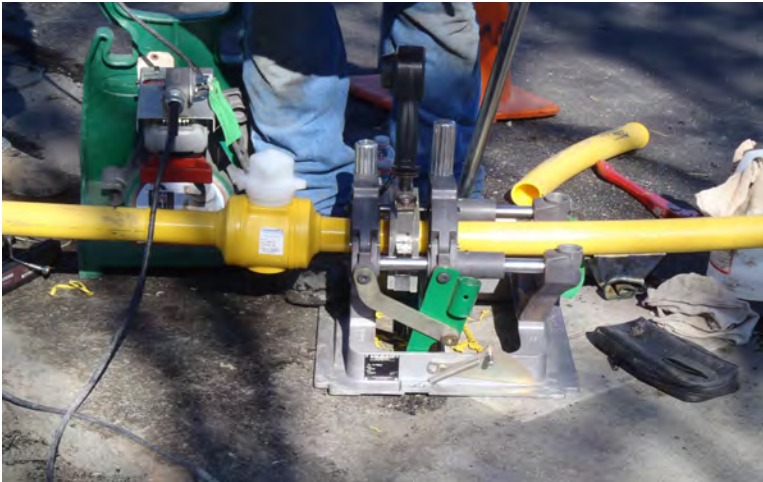
New HDPE gas pipe being fused prior to installation
