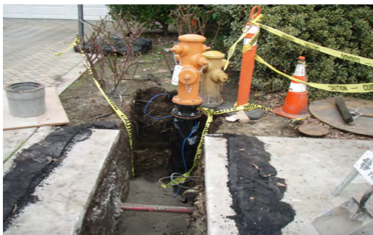
Newly installed fire hydrant service line and assembly on Greenwood Avenue
