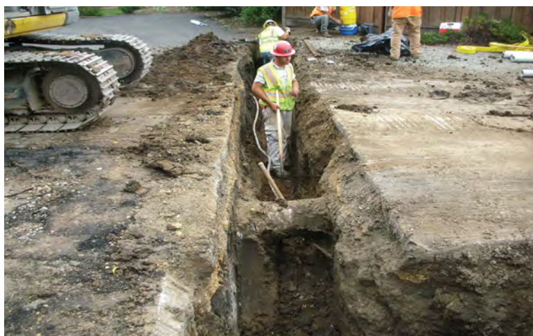
Trenching for installation of HDPE sewer main by open trench method
