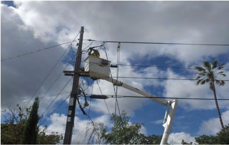
Electric linemen working on overhead electric connection
