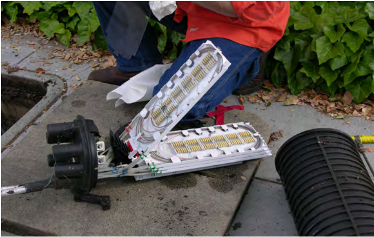
Fiber optic splice closer ready for inspection and work
