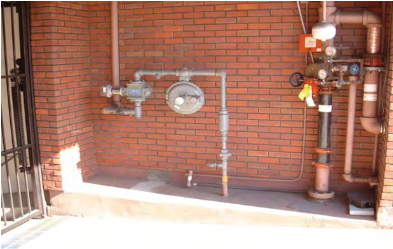
New gas service meter and regulating equipment
