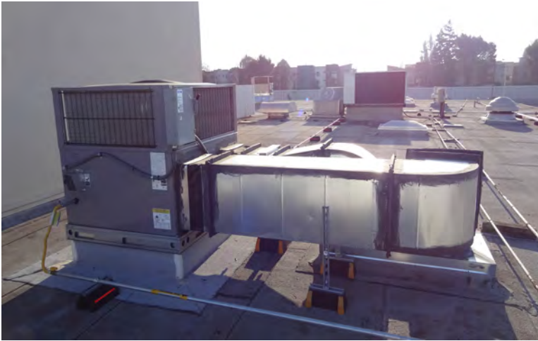
AC gas package unit Municipal Service Center Building C, January 2015
