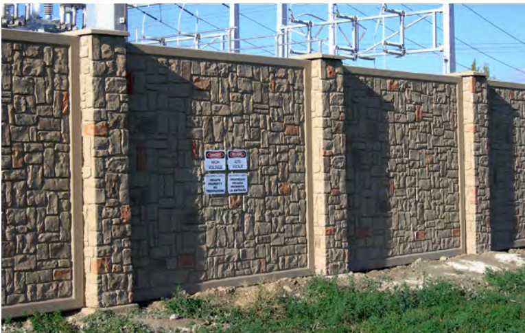
Substation perimeter wall providing security for the enclosed equipment
