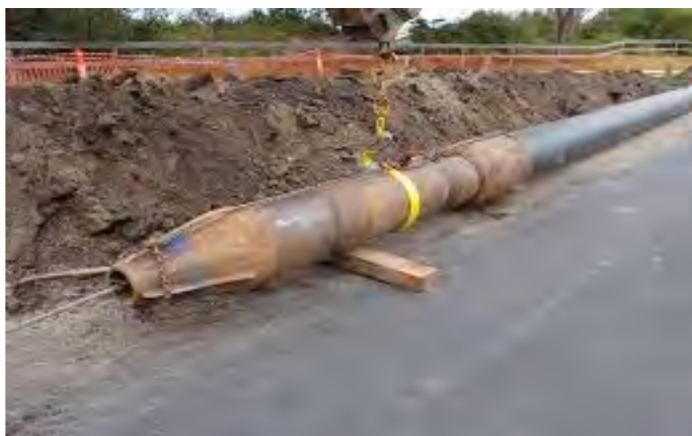
Sewer Main Replacement Project using Pipe Bursting Method
