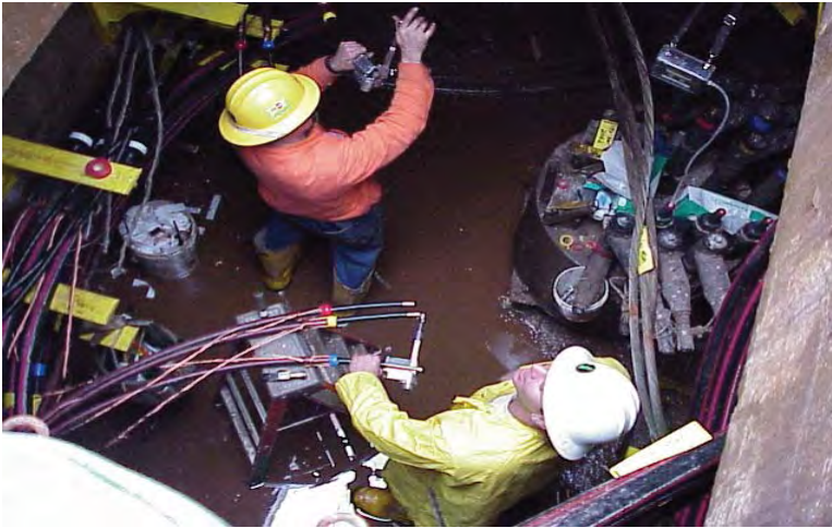
Electric crews working in an underground vault terminating cables
