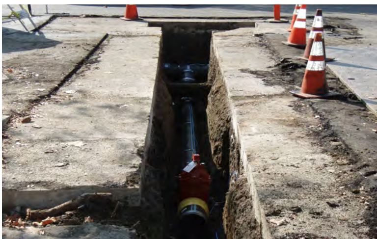
New HDPE main connecting to side street with new valve
