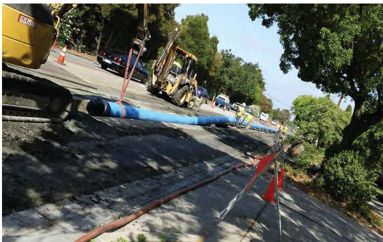
16" HDPE pipe ready to be installed by open trench method
