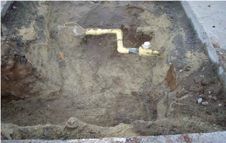
Installation of new HDPE gas service main
