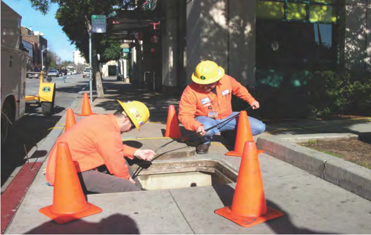
Fiber optic crew installing new fiber optic cables
