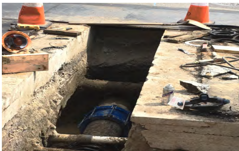
Installed 16" HDPE pipe waiting to be backfilled
