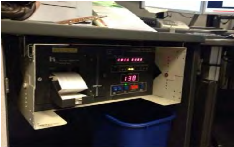
Current Internal Alarm System Control Panel
