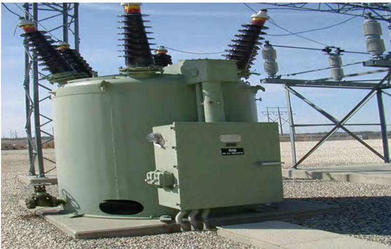
High voltage circuit breakers
