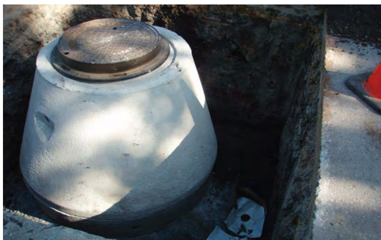
Sewer manhole base
