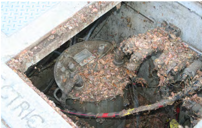
Underground transformer and cable after years of service
