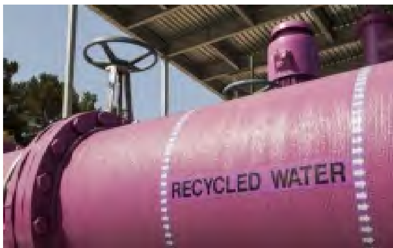
Recycled water piping
