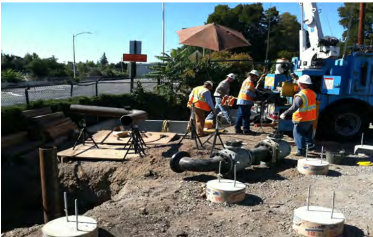
Installation of new HDPE gas service main
