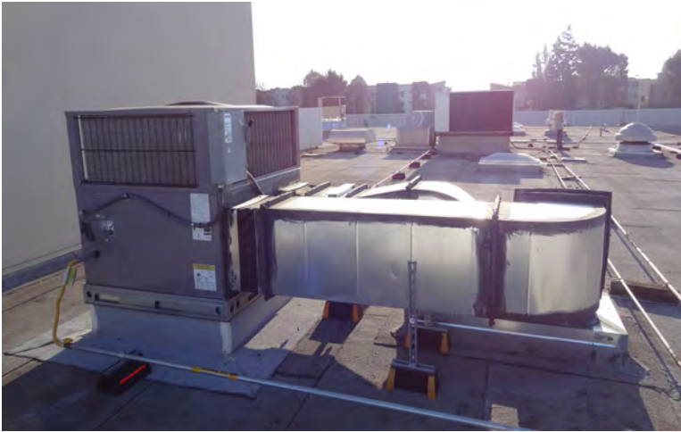
AC gas package unit Municipal Services Center Building C, January 2015
