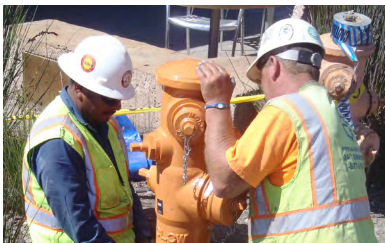
Installation of a new fire hydrant with FlowGuard fire hydrant check valve
