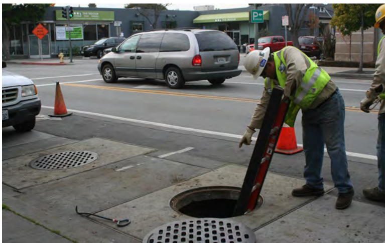
Electric crews preparing to enter underground vault
