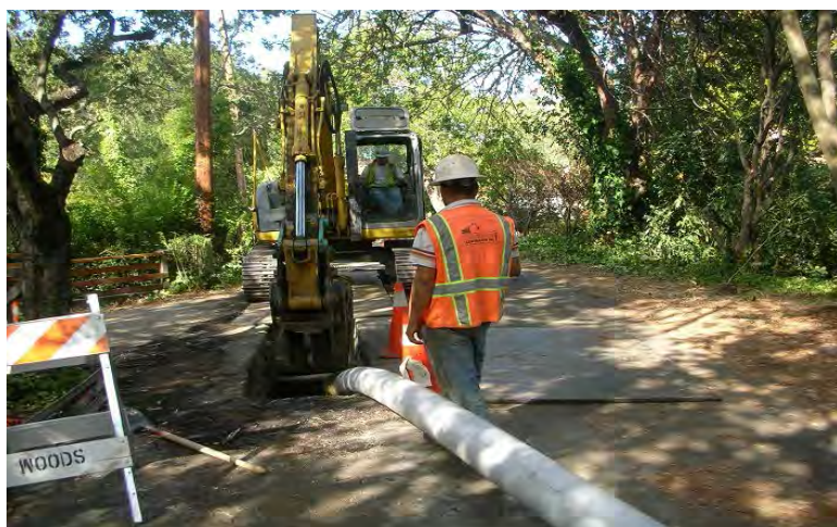
Installation of HDPE sewer main by directional drilling method
