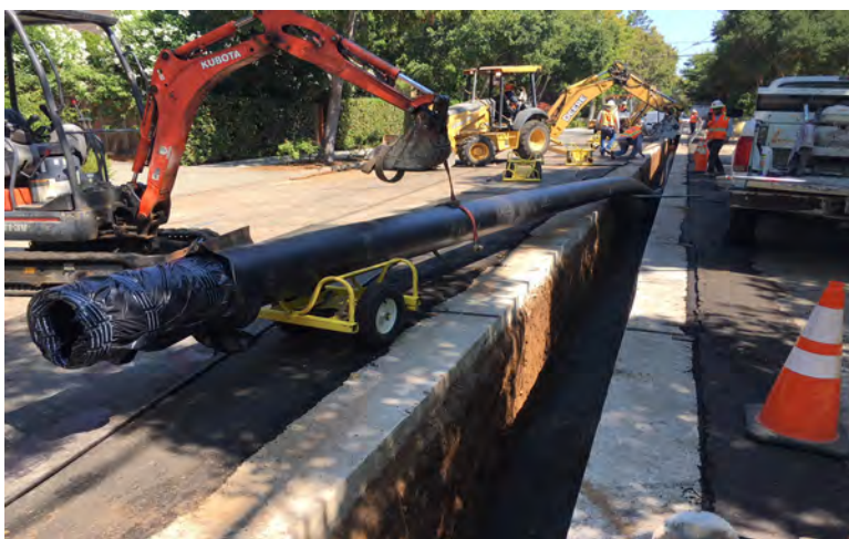
16" HDPE pipe ready to be installed
