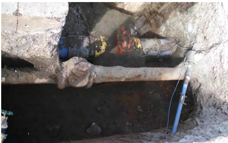
Old Water Main being Replaced
