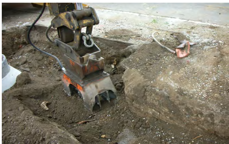
Equipment used to install fuse High Density Polyethylene (HDPE) pipe
