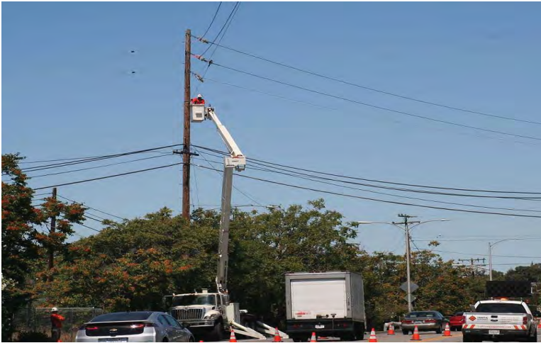
Electric linemen working on 60kV overhead lines
