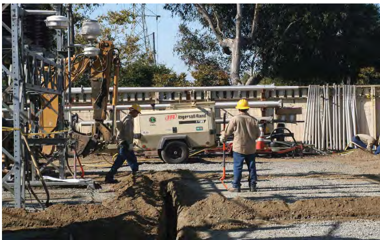
Substation crews installing underground facilities
