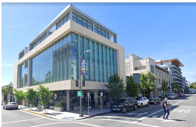
Figure 22: South side of Hamilton Avenue, looking southwest. Source: Google Maps, 2019.
