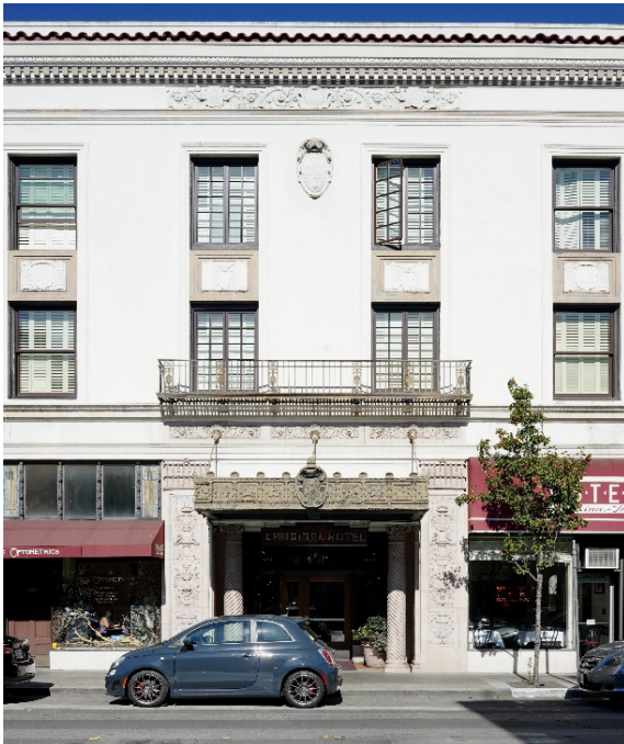
Figure 6: Primary facade, main entrance to hotel.
