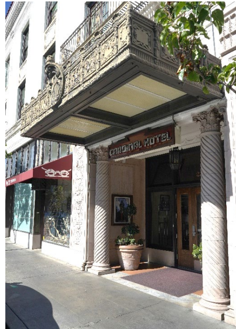
Figure 7: Detail, main entrance to hotel.
