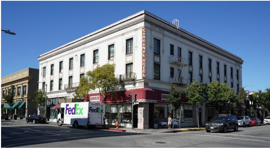
Figure 3: Primary facade (left) and secondary facade (right), looking west
