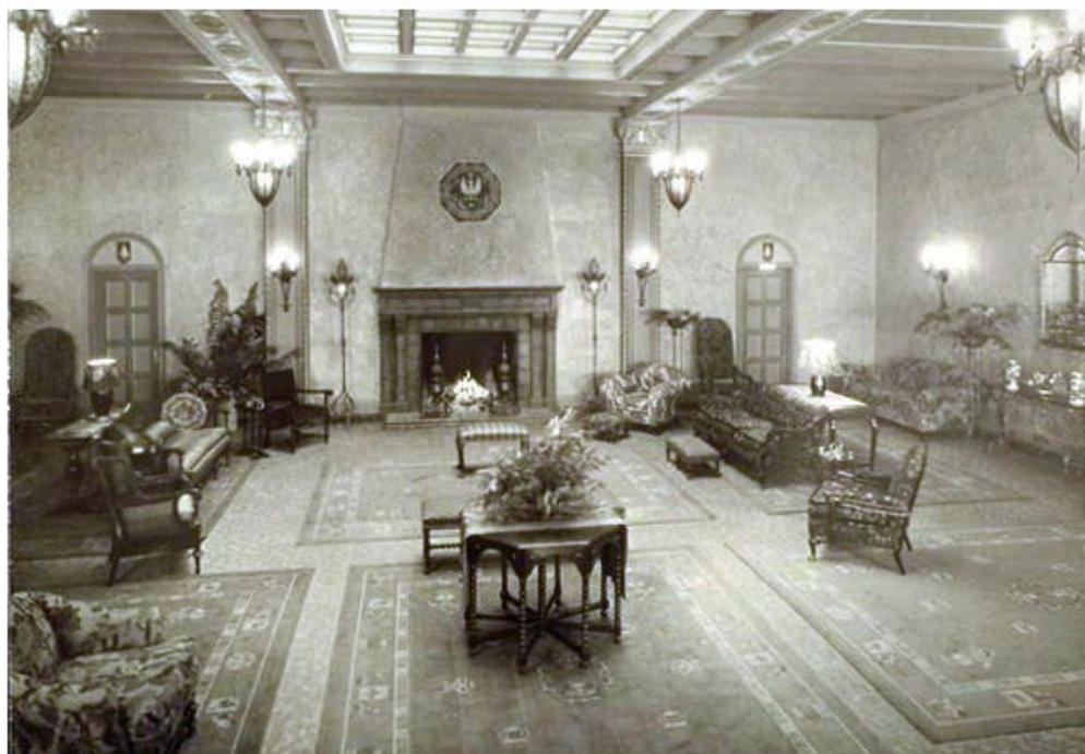
Figure 17: Lobby and lounge, 1924. Source: Palo Alto Historical Association.
