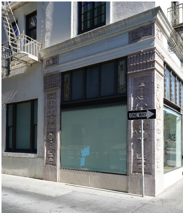
Figure 12: Ground floor, first bay of side (southwest) façade, looking north.
