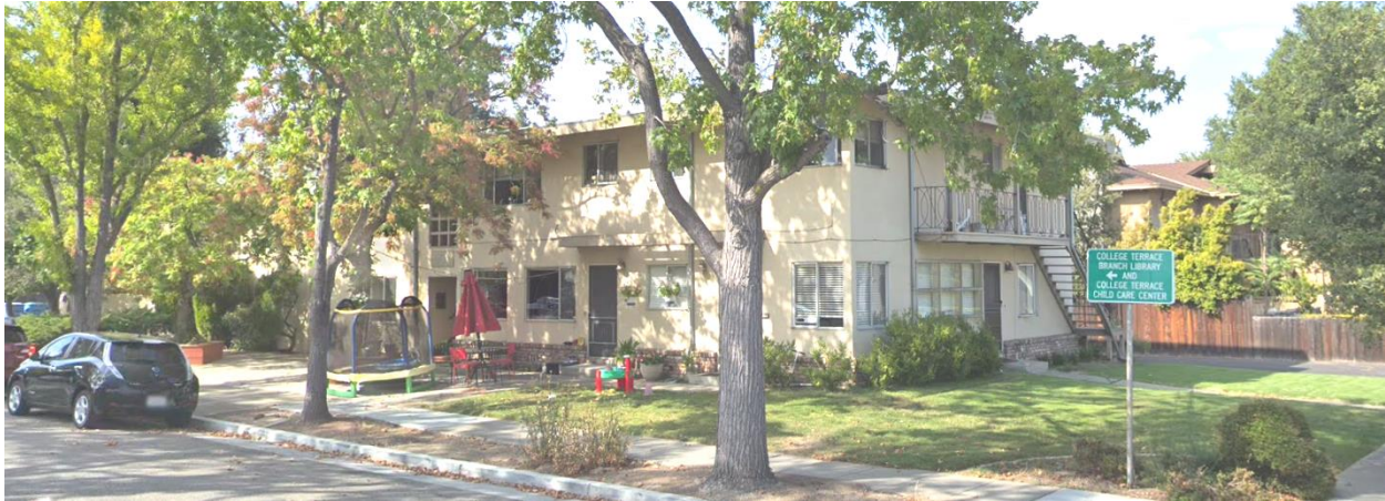
Adjacent Apartment Building
