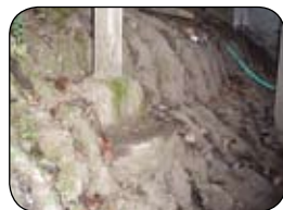
Visible erosion under a deck is common.
