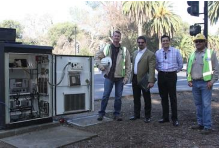
Trafficware CEO, John Newhard (second from left), joins City of Palo Alto staff to turn on the new traffic signal system at the Palm and Arboretum intersection.
