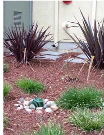
Roof runoff is directed onto landscaping for infiltration in San Jose
