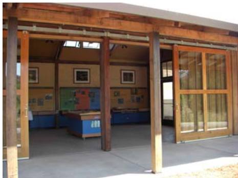
The Arastradero Preserve Interpretive Center was built using straw bale construction, solar panels, and salvaged building materials
