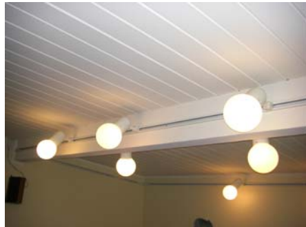
Arthur Keller designed energy efficient dimmable fluorescent light fixtures
