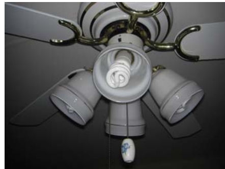
Compact fluorescent bulbs have replaced incandescents
